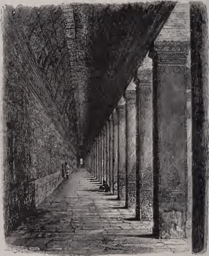
INTERIOR OF WESTERN GALLERY, NAKHON WAT.
